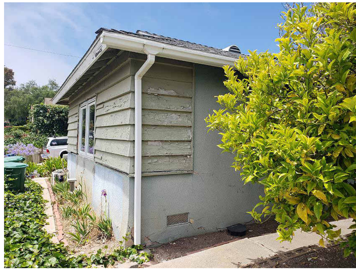
WEST SIDE OF GARAGE
