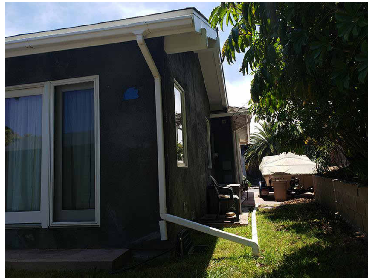
EAST SIDE OF RESIDENCE
