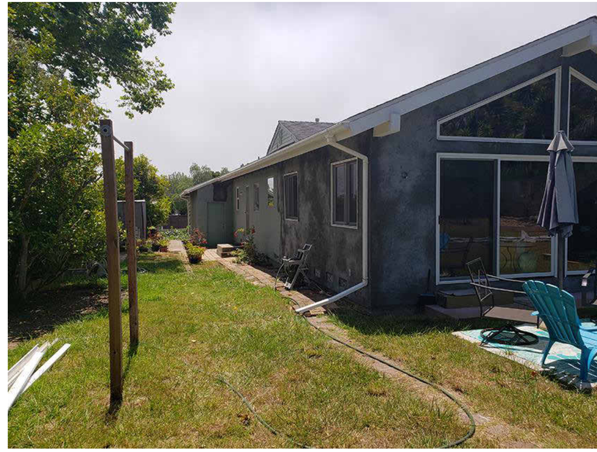
WEST SIDE OF RESIDENCE
