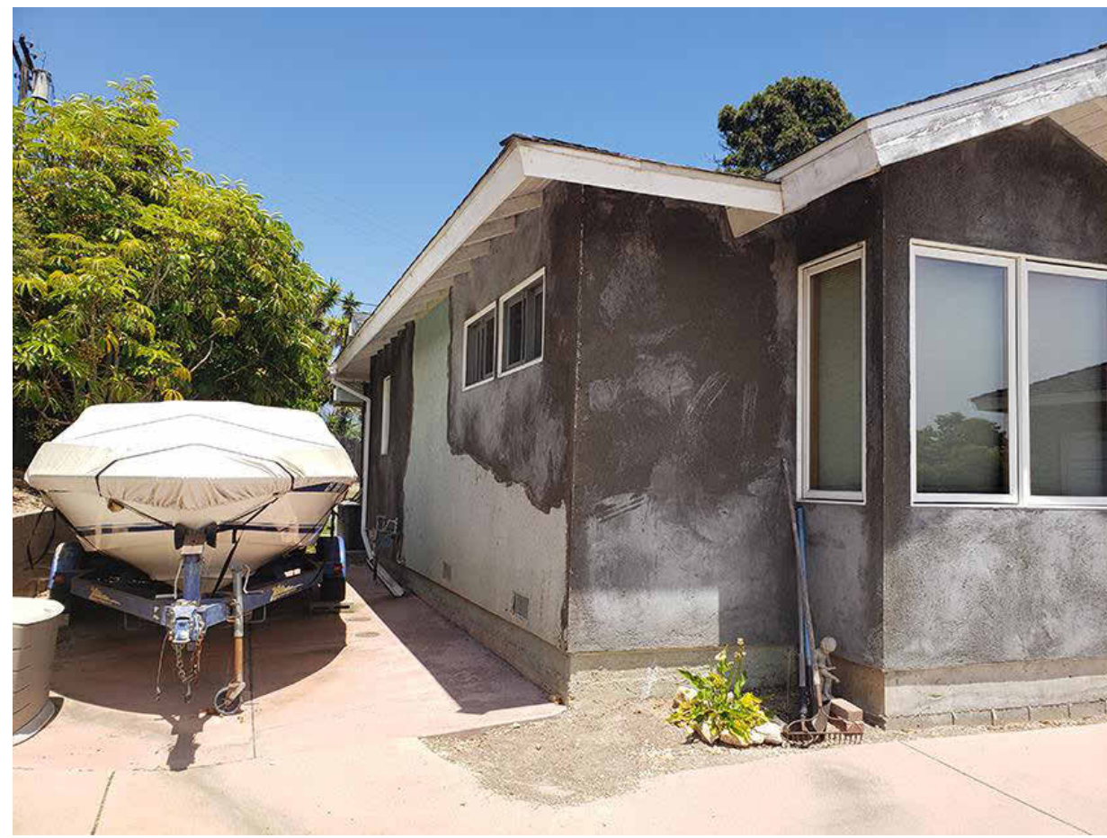
EAST SIDE OF RESIDENCE
